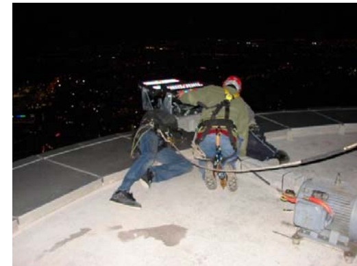
Chris Huff (Modus) and Tony (TRS) installing one of the Color Kinetics Color Reach Luminaires
